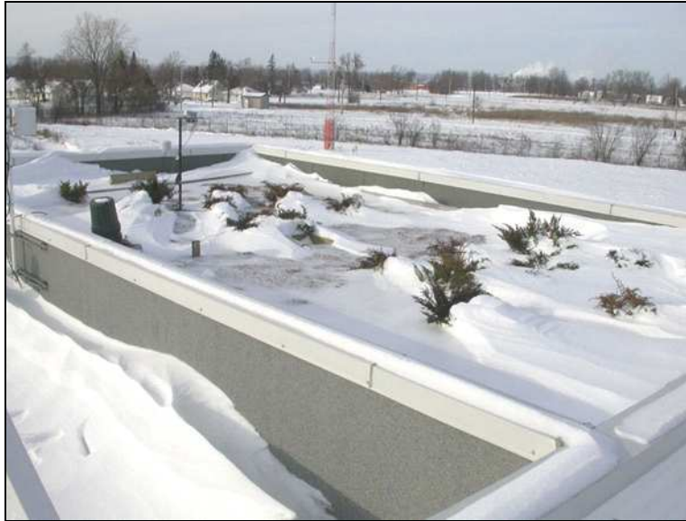
Figure 4.2.2 A green roof during winter
