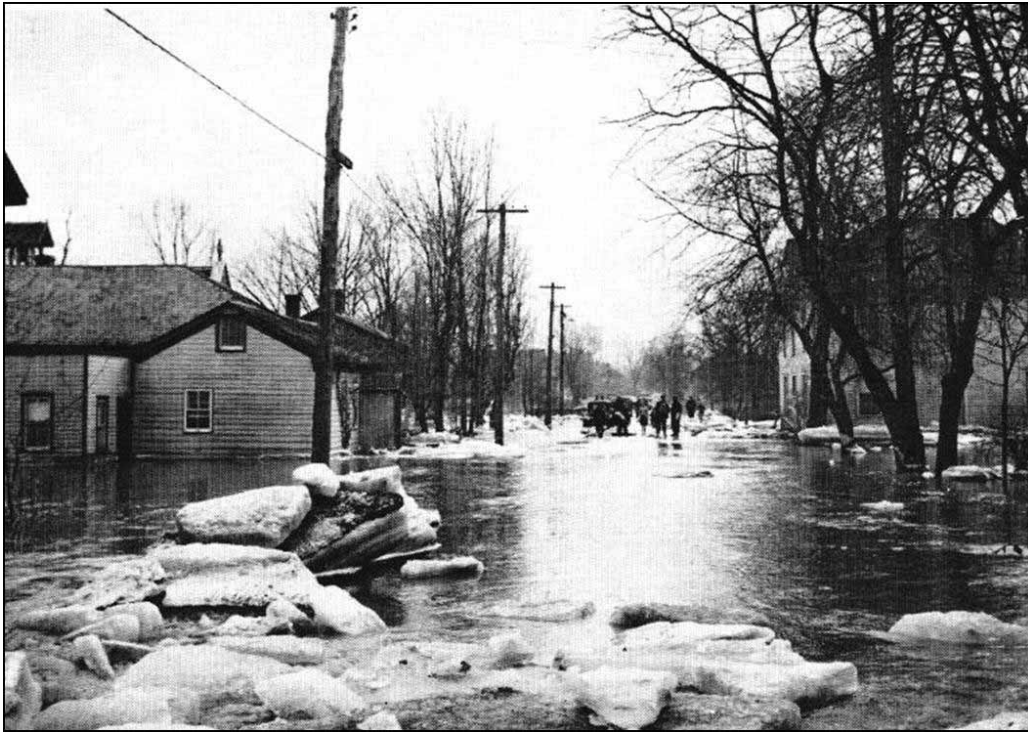
Figure 13: Flooding in Glen Williams, 1946, caused by an ice jam
