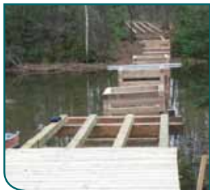
Island Lake boardwalk construction
