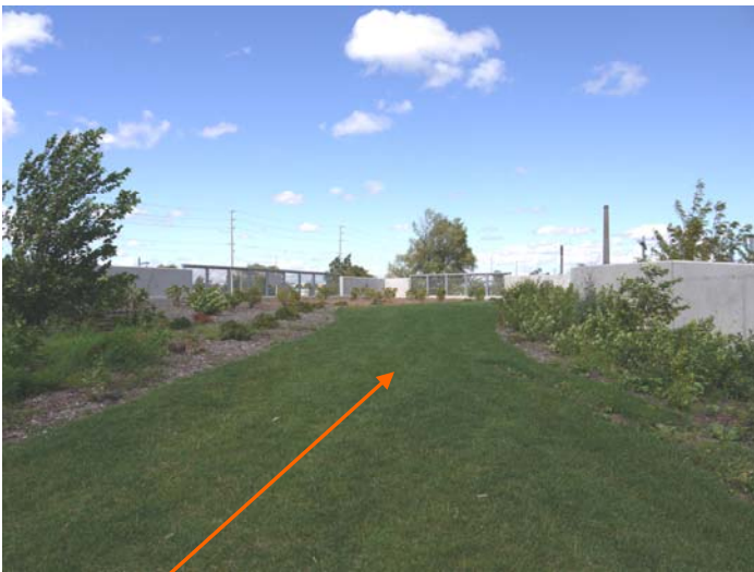
Green Roof is another feature on-site
