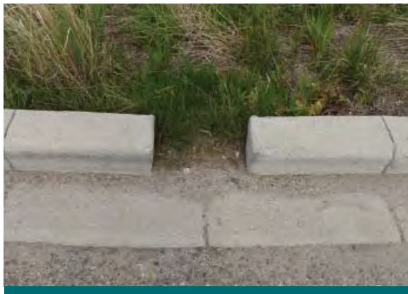
Figure 6.4.1: This notched curb cut at the City of Calgary's City Hall provides flow to a bioretention area from a parking area. More notches may be required to match the inlet capacity of a curb cut. (Source: Aquafor Beech)
