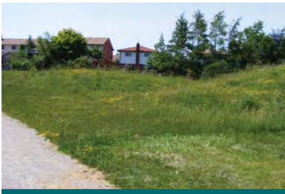
Figure 2.8.3: Micro-grading can create subtle and organic landforms like gently rolling hills that help reduce stormwater runoff. (Source: Aquafor Beech)
