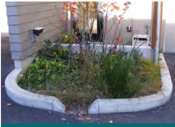
Figure 6.4.5: A standard curb cut is a simple yet effective means of providing drainage and protection. (Source: Aquafor Beech)
