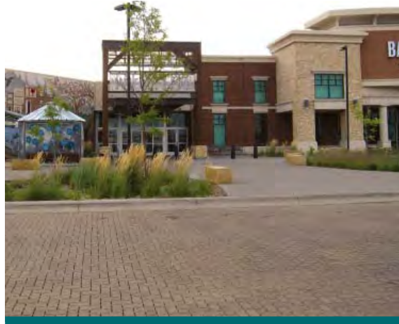
Figure 2.2.3: Permeable pavers come in a variety of shapes and sizes. They can be arranged in patterns that enhance site aesthetics. Here permeable pavers are used to mark a pedestrian crossing zone at a mall entrance. (Source: CVC)
