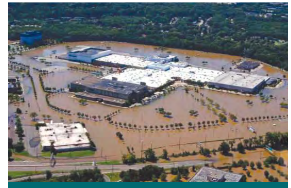
Figure 11.0.2: This shopping centre was forced to temporarily shut down due to significant urban flooding. In addition to lost business, flooding can result in the loss of goods. Improving drainage and reducing the amount of impervious surface could help alleviate urban flooding in this area. (Source: CVC)
