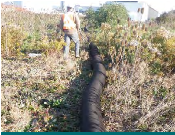
Figure 9.6.2: A filter sock installed at the IMAX Project site as part of the erosion and sedimentation control plan. (Source: Aquafor Beech)
