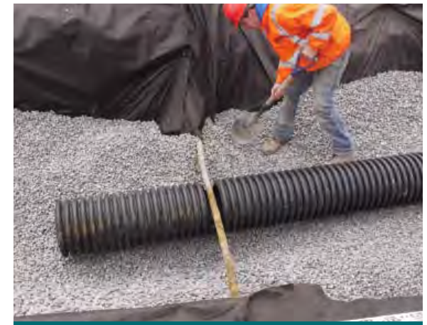
Figure 9.4.2: The construction team cuts a notch a perforated pipe to accommodate a gas line. (Source: Aquafor Beech)
