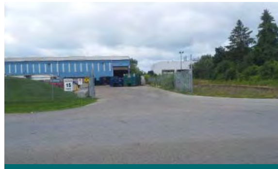
Figure 4.7.1: Here a loading bay and waste storage area drain to the road. P2 practices could improve runoff quality from this site. (Source: Aquafor Beech)
