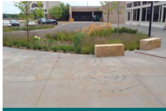
Figure 4.4.1: Large pedestrian areas, such as mall entrances, are ideal targets for LID retrofits. (Source: CVC)
