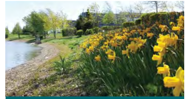
Figure 10.1.1: At this stormwater management facility, a municipal-private partnership approach to maintenance was established. The municipality is responsible for life-cycle activities that are critical to maintaining the facility, including outlet inspections and dredging. The land management company that owns the adjacent property is responsible for maintaining landscape features. (Source: CVC)
