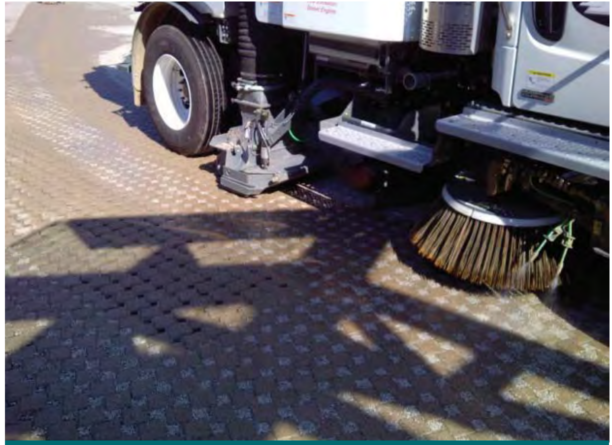
Figure 10.2.5: Vacuum sweepers will remove accumulated debris between block pavers, but can also remove aggregate from paver joints (note the voids behind the sweeper truck). Always replenish any lost joint aggregate following vacuum sweeping. (Source: Aquafor Beech)
