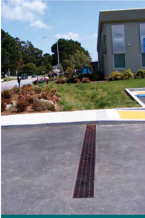
Figure 6.4.7: Grated strip drains ensure onsite control at parking lot entrances. (Source: Aquafor Beech)
