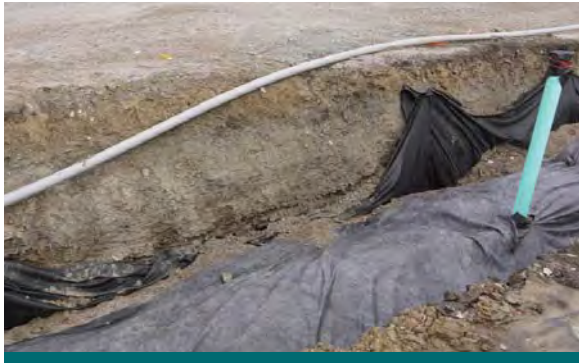
Figure 9.6.1: Infiltration areas are covered with sacrificial strips of geotextile when filled with media to protect them from contamination. Contractors can then clean out debris without affecting the infiltration area. (Source: CVC)
