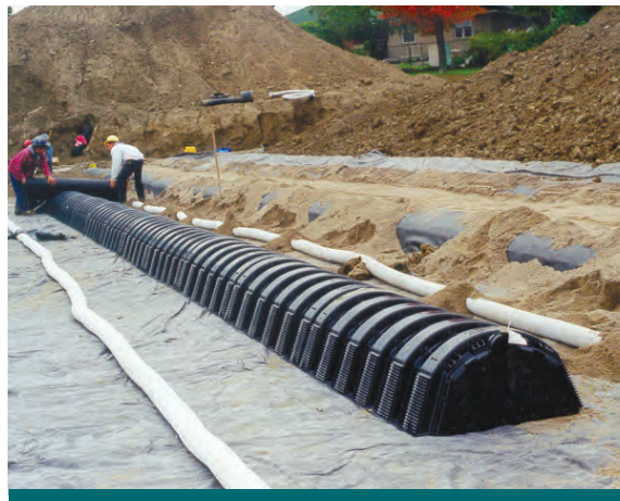
Figure 2.5.2: Infiltration chamber retrofits require significant excavation. (Source: Aquafor Beech)
