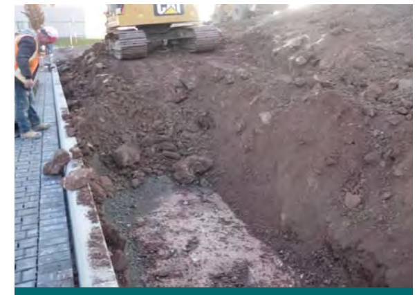
Figure 9.2.4: The granular base has been removed from the perforated pipe area. (Source: Aquafor Beech)
