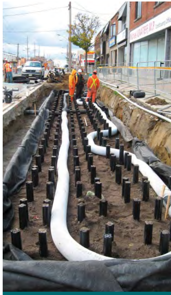
Figure 2.9.3: During installation of a soil support system, significant excavation will be required. Modular units allow for design flexibility, such as this long configuration. (Source: DeepRoot)
