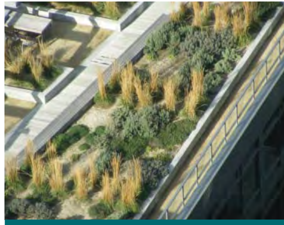
Figure 2.10.2: High-rise condominiums represent excellent opportunities for green roofs due to their large flat rooftops and the opportunity to create amenity space for residents. (Source: Aquafor Beech)
