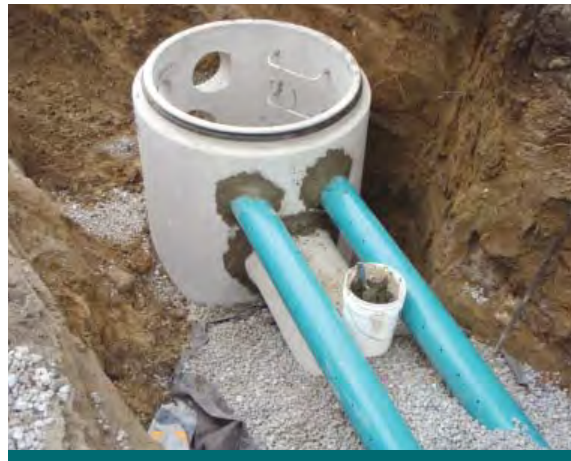
Figure 2.6.2: Perforated pipe systems employ many of the same materials and construction practices as conventional storm sewer pipes. Note the perforations in the blue pipe. (Source: Aquafor Beech)
