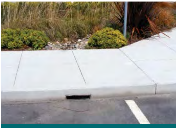
Figure 6.4.4: The covered curb inlet is a common feature of conventional and LID designs. (Source: Aquafor Beech)
