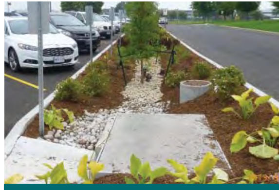
Figure 2.3.2: This parking lot bioretention area treats runoff from a conventional asphalt parking lot. It incorporates additional proprietary stormwater treatment devices within the bioretention to provide even greater water quality treatment. (Source: CVC)
