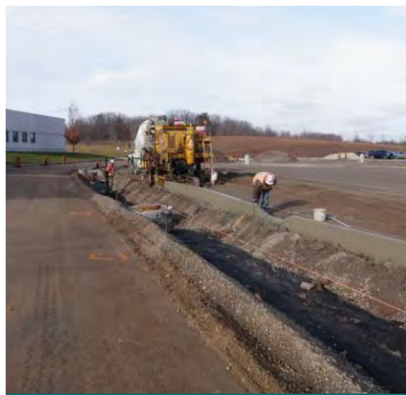
Figure 6.4.25: The bioswale and new curbing being installed at the IMAX Project. (Source: Aquafor Beech)
