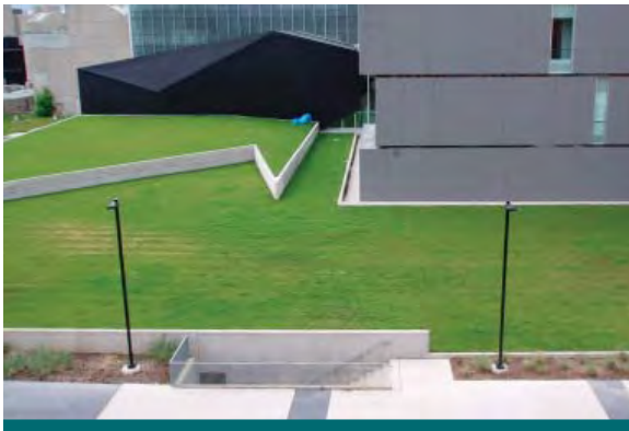
Figure 2.10.1: Green roofs can also be incorporated in other types of structures. In this case a green roof (turf) was installed on top of a parking garage.
