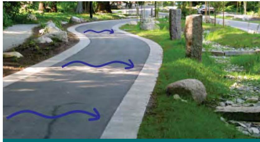
Figure 6.4.3: Flush curbs on both sides of this street allow for drainage from left to the bioswale on the right. (Source: City of Vancouver)
