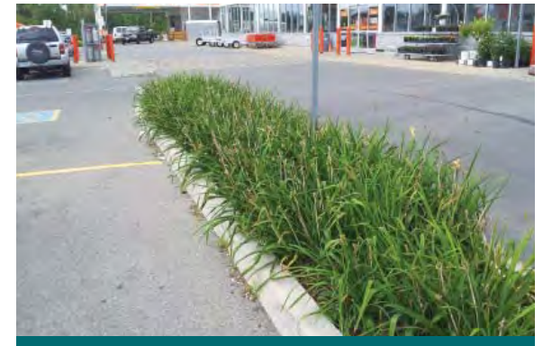
Figure 4.4.2: Look for existing features that can be modified to include LID practices without compromising site function. This parking lot island is an ideal location for a bioretention planter. (Source Aquafor Beech)
