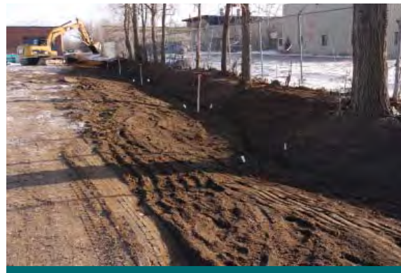
Figure 2.8.4: During the Bernardi retrofit the buffer strips were excavated and compacted topsoils were disposed. (Source: Aquafor Beech)
