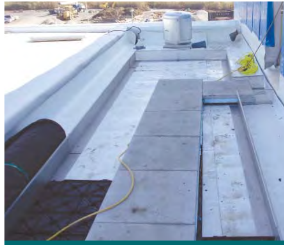
Figure 9.5.2: Contractors installed planks to avoid walking on delicate roofing components. (Source: CVC)
